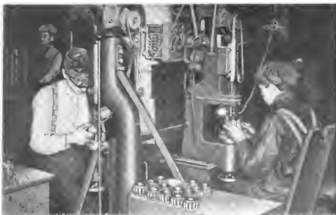
RIVETING THE CAGE RING STUDS HOLDING THE ROLLERS.
